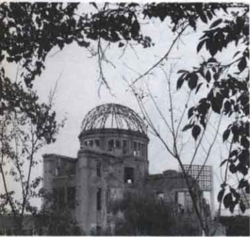
The remains of a building at the hypocenter of the Hiroshima explosion; the bomb exploded 500 meters above it. This is the only building in the area to survive, even in part.
